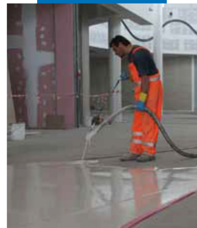
Mechanical application of Ultratop
