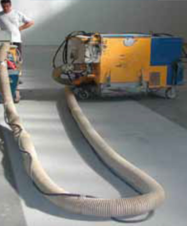
Preparation of the substrate by shot-blasting
