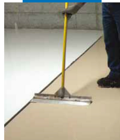
Smoothing Ultratop immediately after spreading
